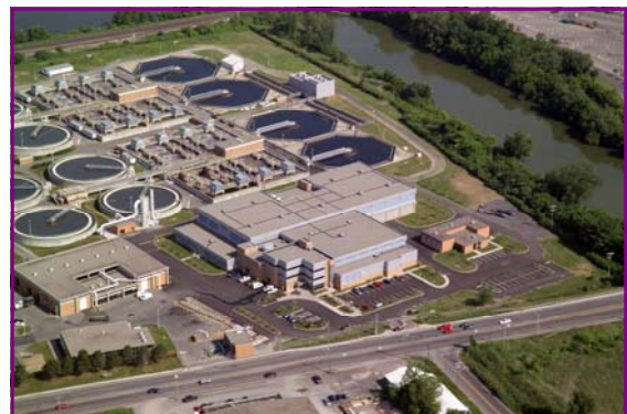
Metropolitan Syracuse Wastewater Treatment Plant (Metro) on Hiawatha Boulevard.
