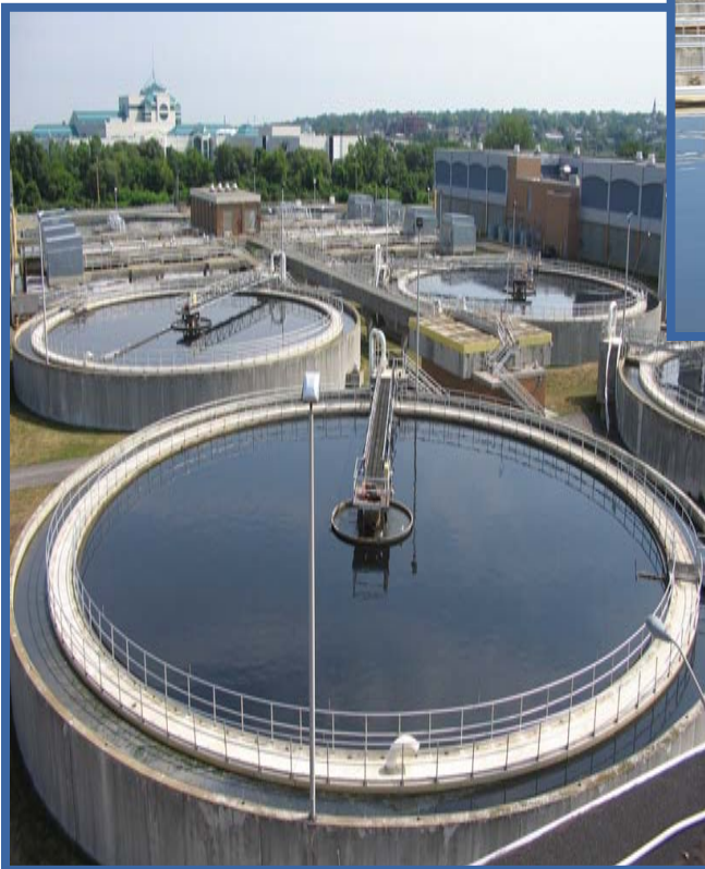
Primary Clarifier Tanks
