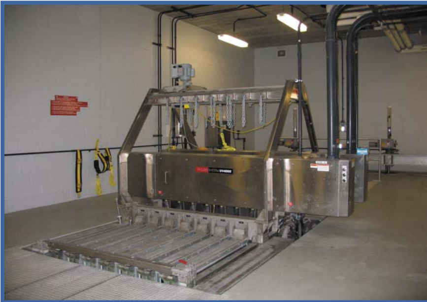
Trojan UV 4000 Disinfection Unit
