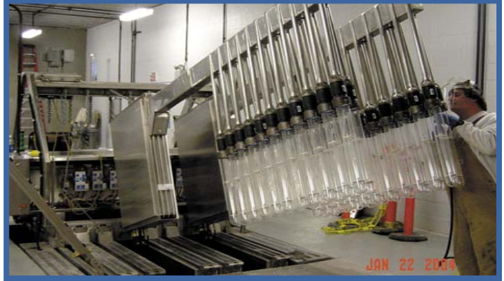
Installation of UV Disinfection Lights
