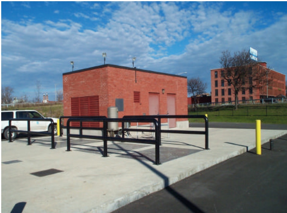
Butternut Floatables Control Facility
