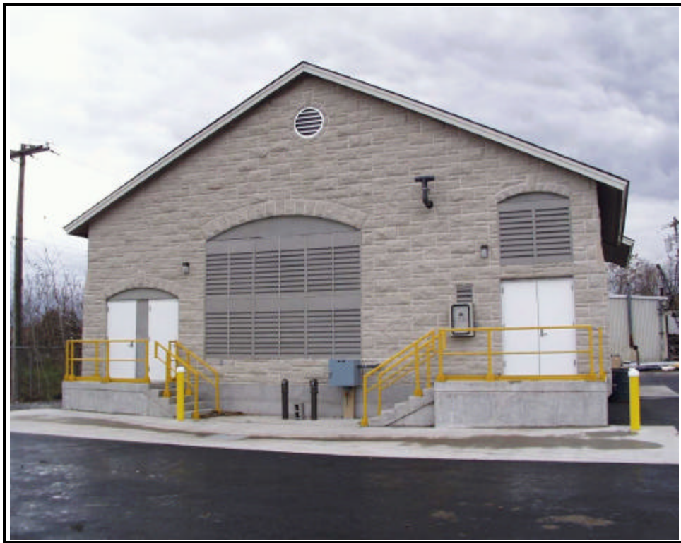
Kirkpatrick Pump Station Upgrade
