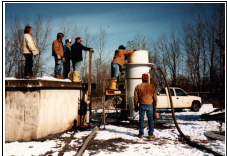
Davis Road Pump Station, Force Main Cleaning
