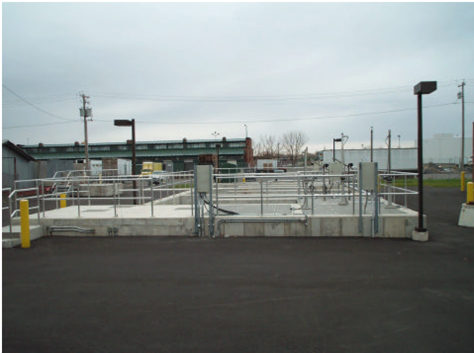
Hiawatha RTF, Disinfection Tank
