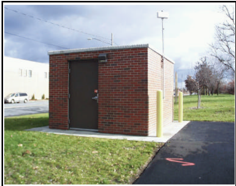
Erie Boulevard Storage System, Control Building
