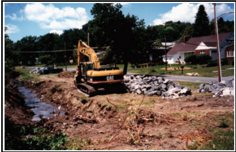
Meadowbrook Drainage District Improvements, 2002
