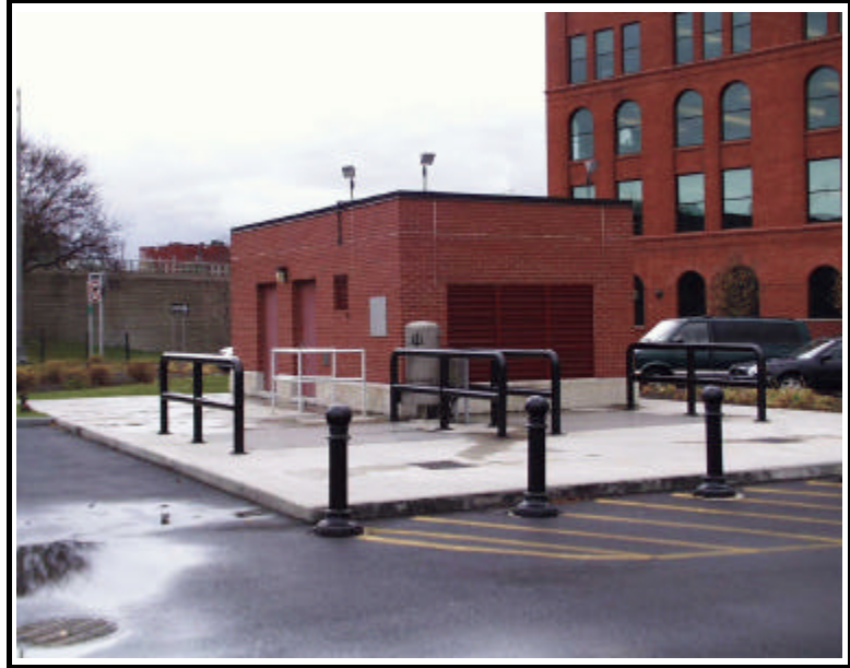
Butternut Floatable Control Facility
