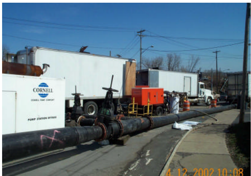
Picture 10 – Bypass pumping operations for rehabilitation of Genesee Trunk Sewer
