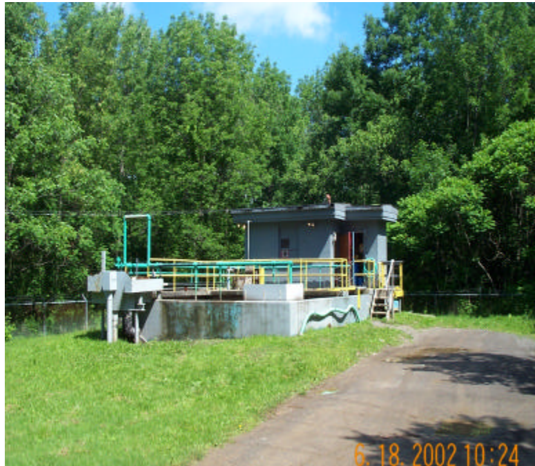
Picture 14 – Existing Harbour Heights WWTP, to be decommissioned
