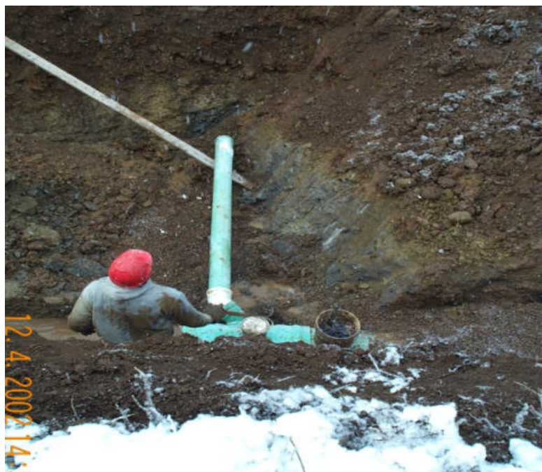
Picture 15 – New sanitary sewer installation for Harbour Heights project
