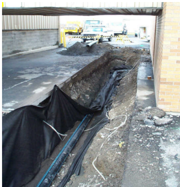
Picture 8 – Installation of new potable water line at Metro WWTP
