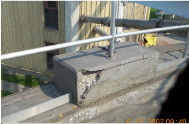
Picture 1 – Metro WWTP Digester No. 2 roof prior to repair
