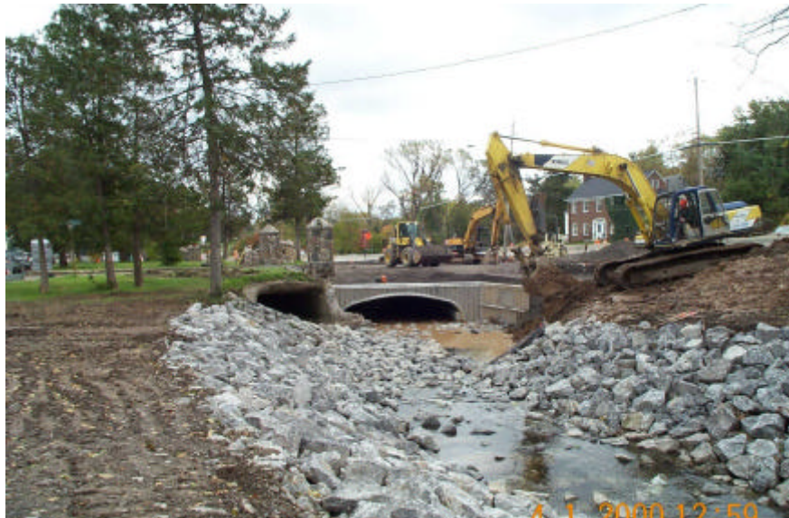
Picture 16 – Installation of new culvert system for Meadow Brook Channel project
