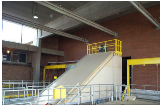
Picture 5 – New FRP cover system for Metro WWTP NSG drywell
