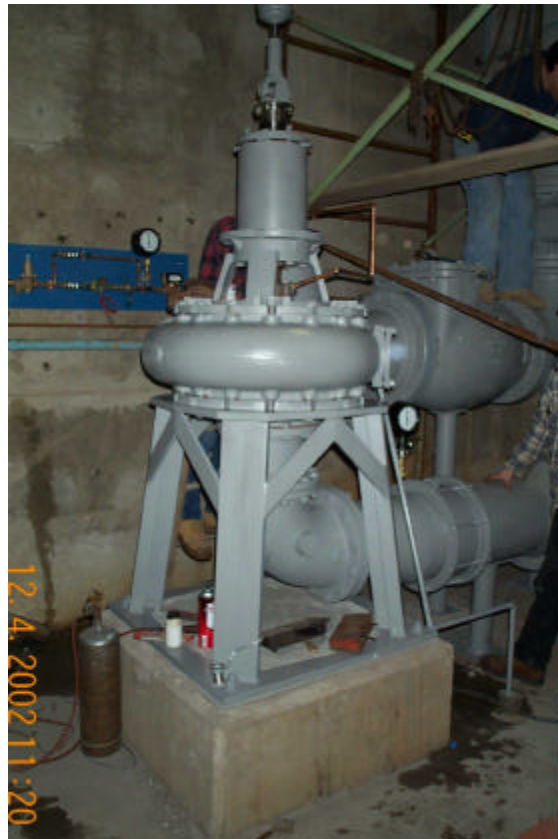
Picture 17 – New pump installation for VFD project
