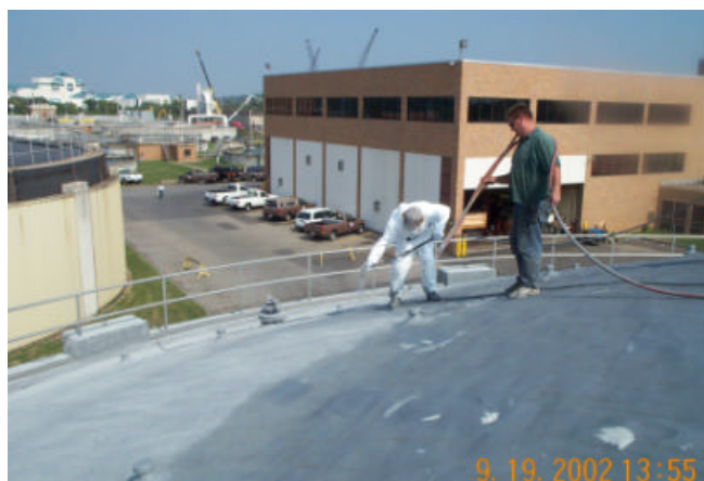
Picture 3 – Application of new roofing system for Metro WWTP Digester No. 2
