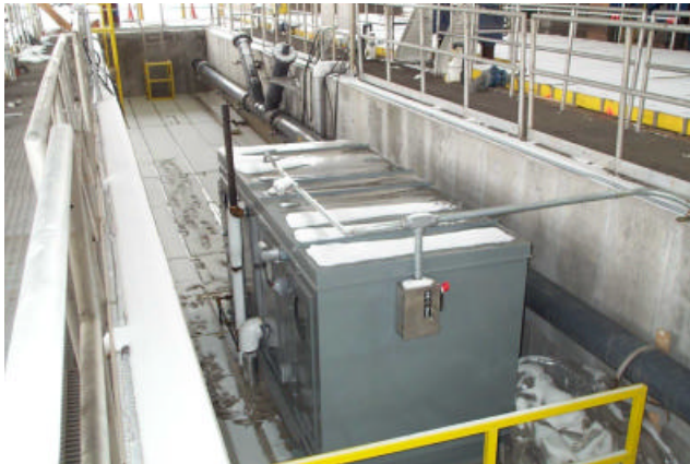
Picture 4 – New H & V unit for Metro WWTP NSG drywell
