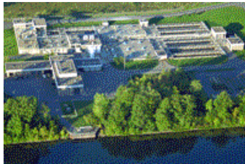
Figure 1.1, Baldwinsville waste water treatment plant
