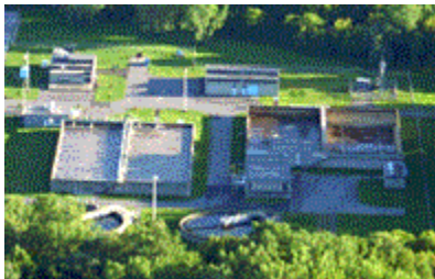
Figure 2.6, Meadowbrook-Limestone waste water treatment plant
