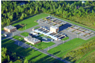
Figure 1.2, Brewerton waste water treatment plant
