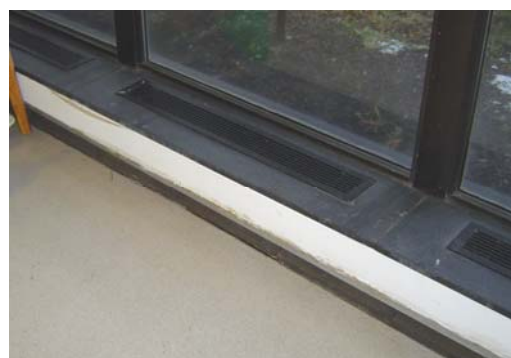
Figure 2.12, Perimeter radiant heat
