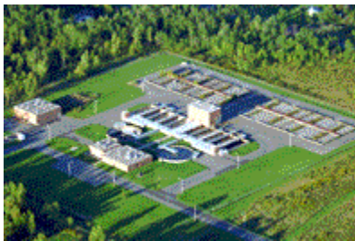
Figure 2.4, Brewerton waste water treatment plant
