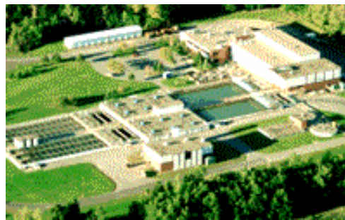
Figure 1.4, Oak Orchard waste water treatment plant
