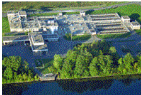
Figure 2.1, Baldwinsville waste water treatment plant
