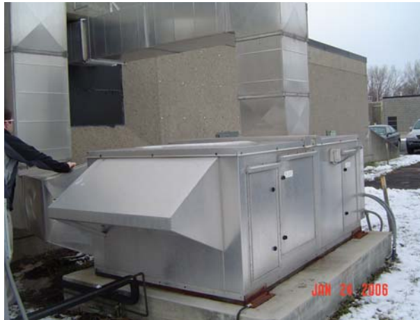
Figure 2.7, Split system serving the office
