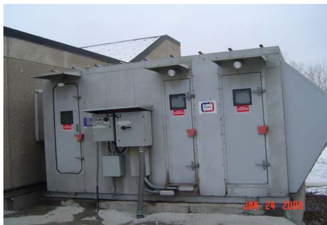
Figure 2.8, Make-Up air unit serving the effluent room
