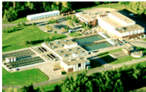
Figure 2.10, Oak Orchard waste water treatment plant
