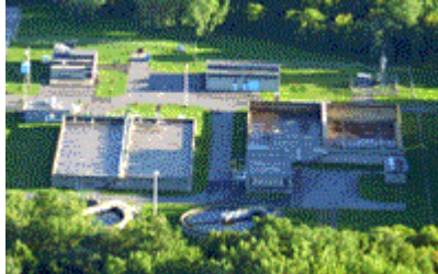
Figure 1.3, Meadowbrook-Limestone waste water treatment plant
