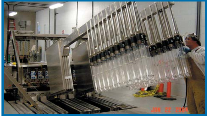
Installation of UV Disinfection Lights
