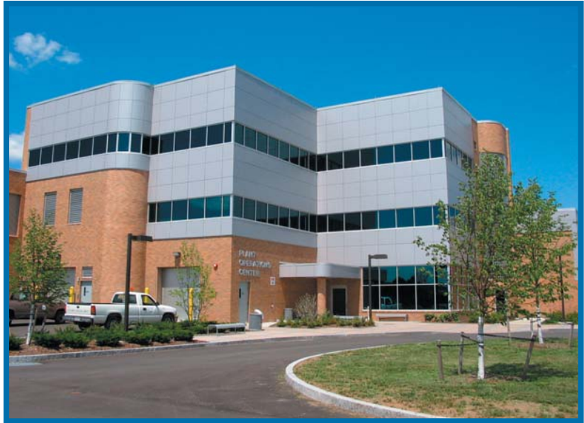
Plant Operations Center
