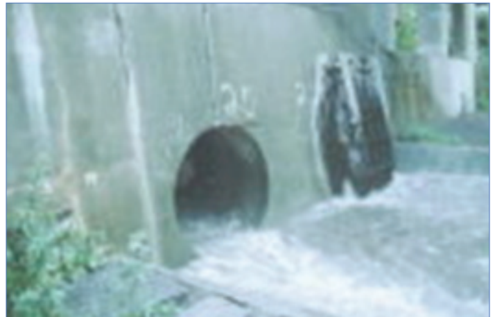
Combined sewer overflow to Onondaga Creek during an intense rain storm, Syracuse, NY
