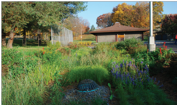
Sunnycrest's rain garden diverts rainwater to the soil, reducing the volume of water entering storm sewers.
