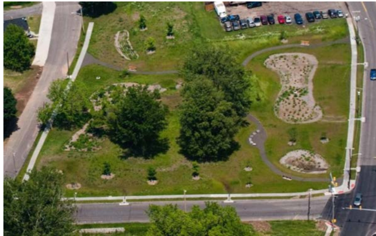
Green Infrastructure Facility Installed on a Two Acre Parcel of Land at the Intersection of Amy Street, Delaware Avenue and Grand Avenue.
