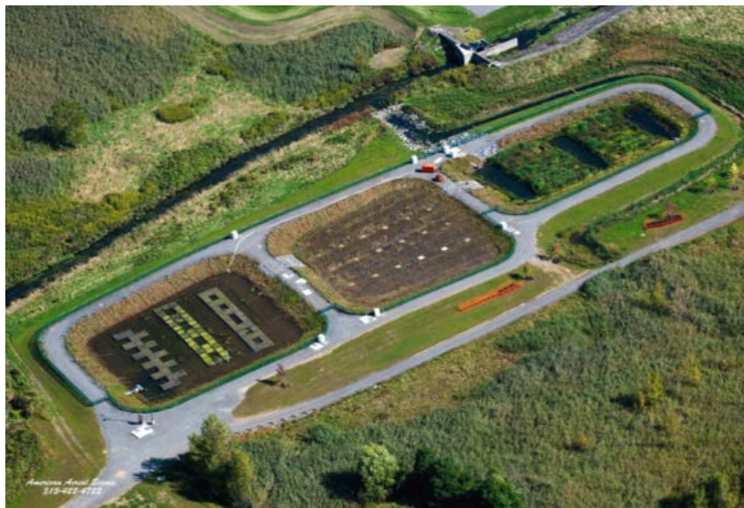
Aerial View of the Harbor Brook Wetland Pilot Treatment System at CSO 018.
