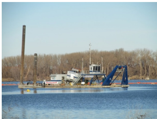
Onondaga Lake Dredging Operations.
