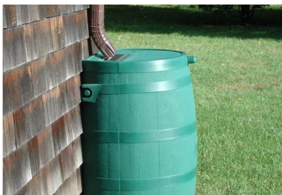
Rain Barrel Installation.
