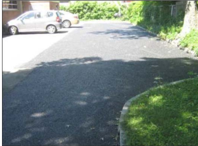
Petit Library Porous Pavement Parking Lot.
