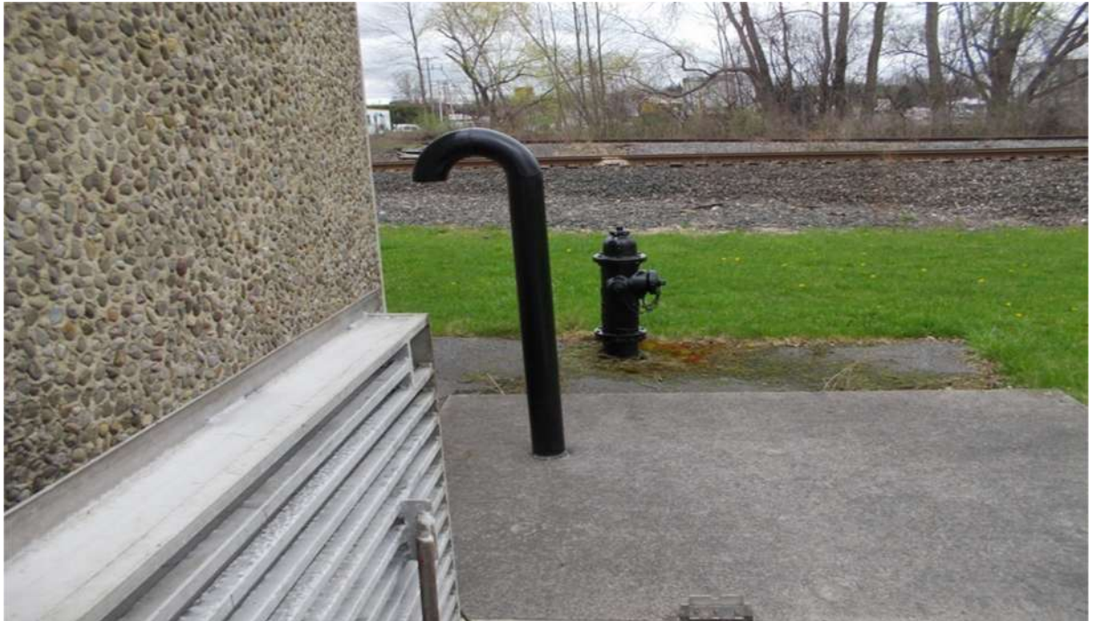
Cane Vent and Bypass Hydrant
