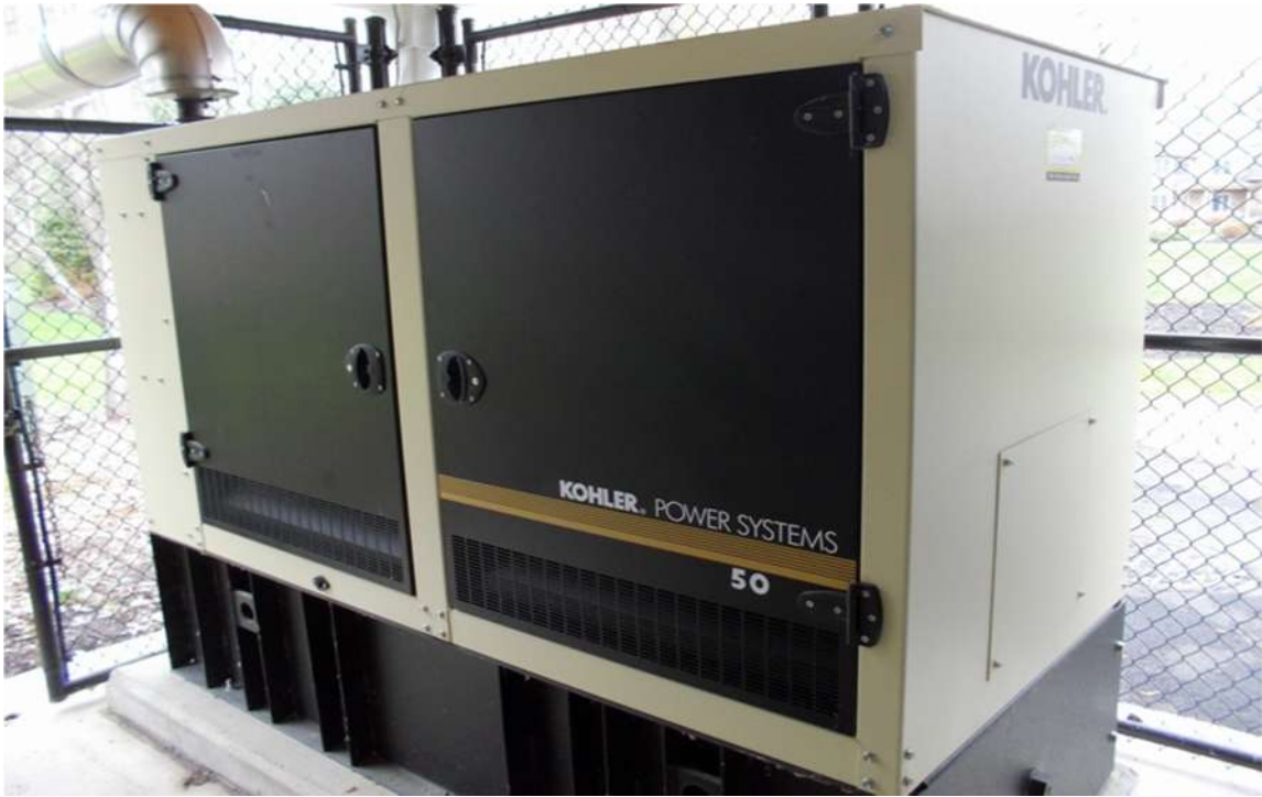
Generator and Control Panels
