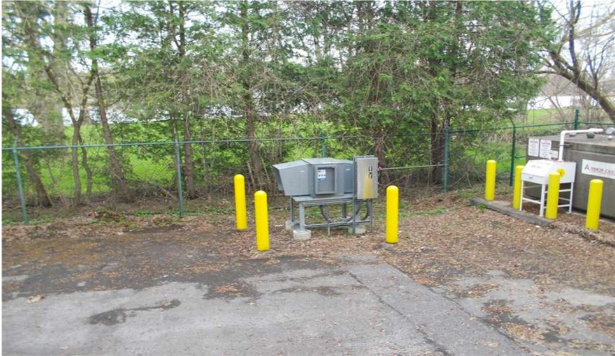
Bollards Protect Hydrant, Vent, Controls
