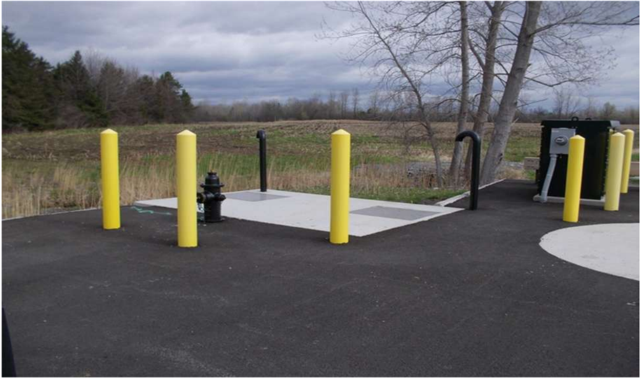
Bollards Protect Hydrant, Vent, Controls
