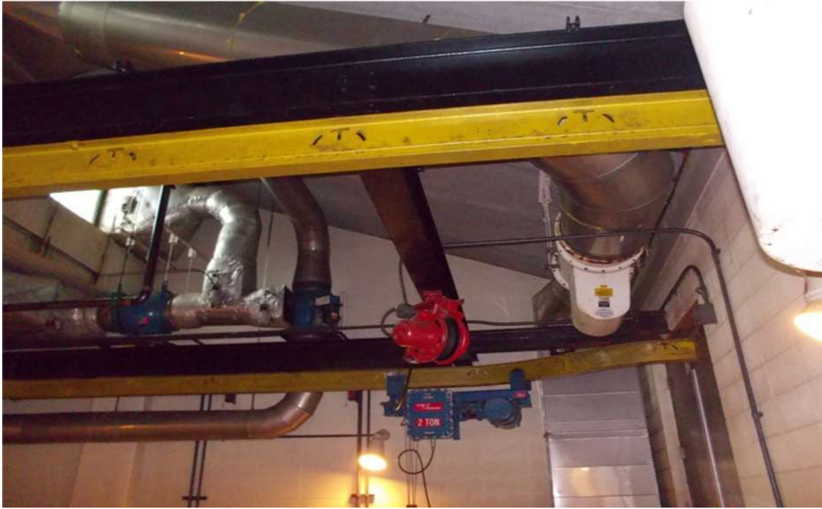
Overhead Crane System
