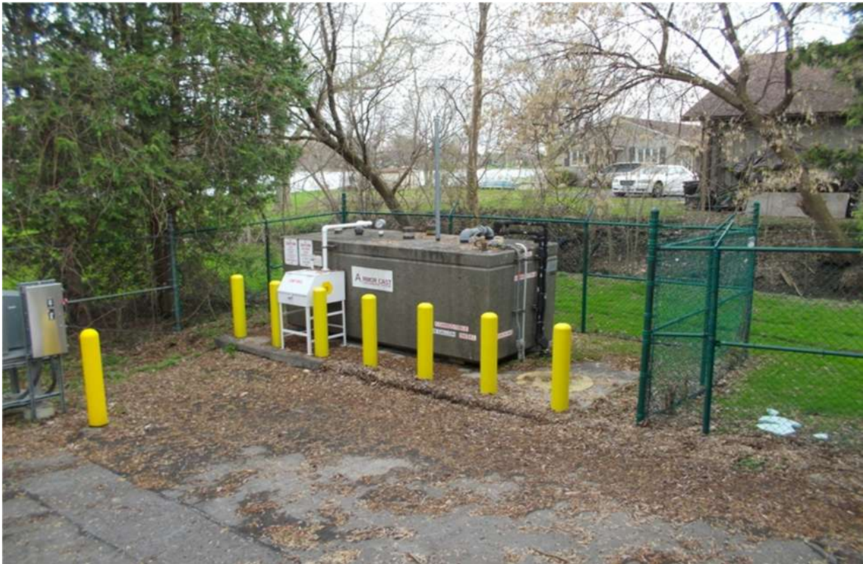
Generator and Fuel Containment
