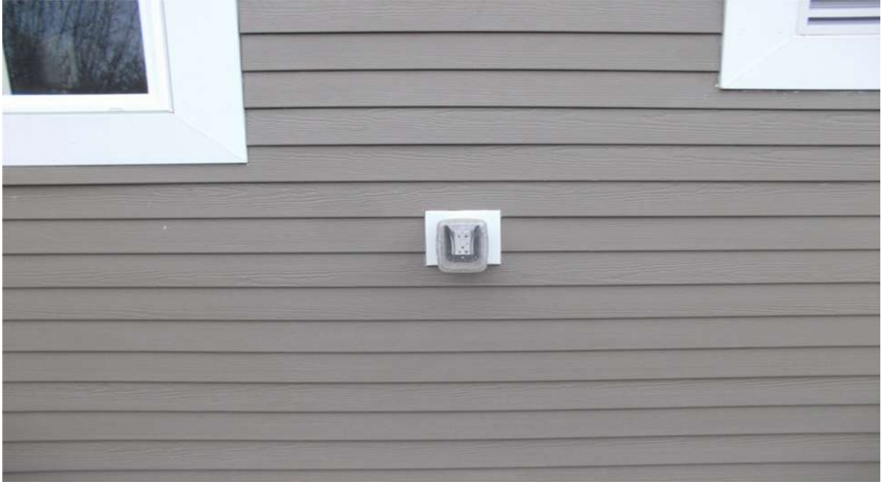
Exterior Power Supply
