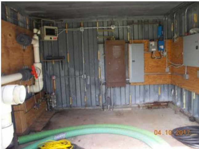
Center-Inside Newell RTF Control Building
