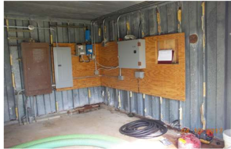
Right-Inside Newell RTF Control Building
