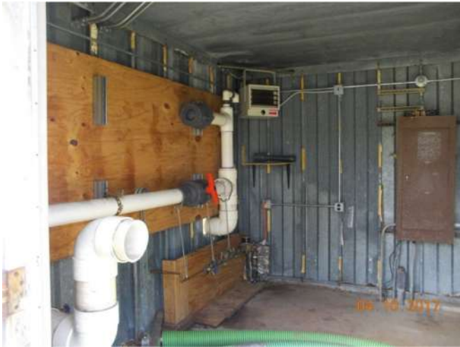
Left-Inside Newell RTF Control Building
