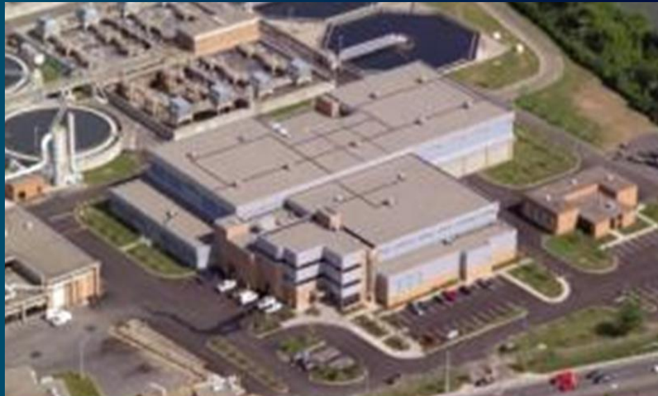
Syracuse Metropolitan WWTP
