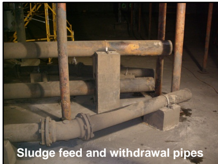
Sludge feed and withdrawal pipes and supports
