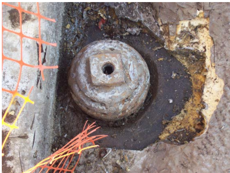
Roof Drain Strainer
