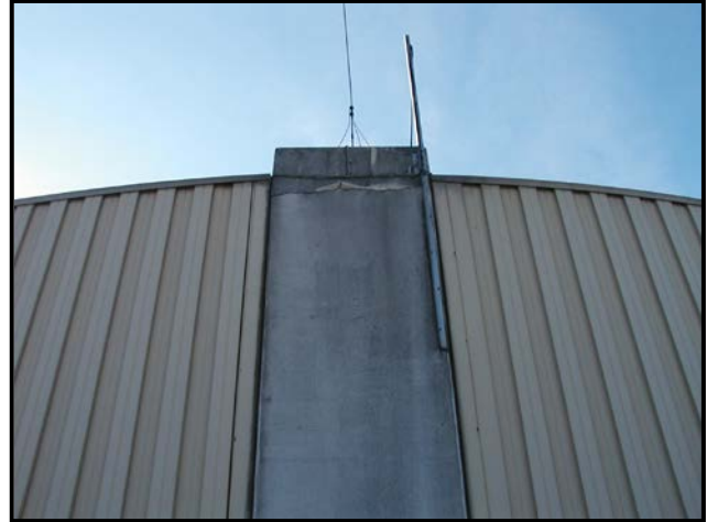
Photo 2: Typical Pilaster (Exterior)
