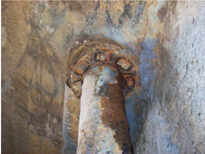
Interior Roof Drain
