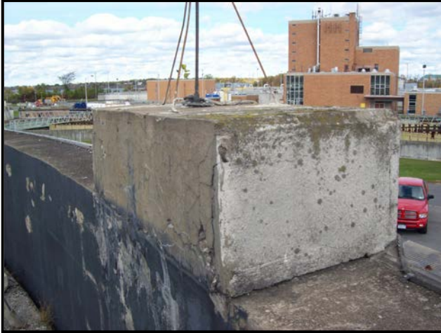
Photo 1: Typical Pilaster (Interior)
