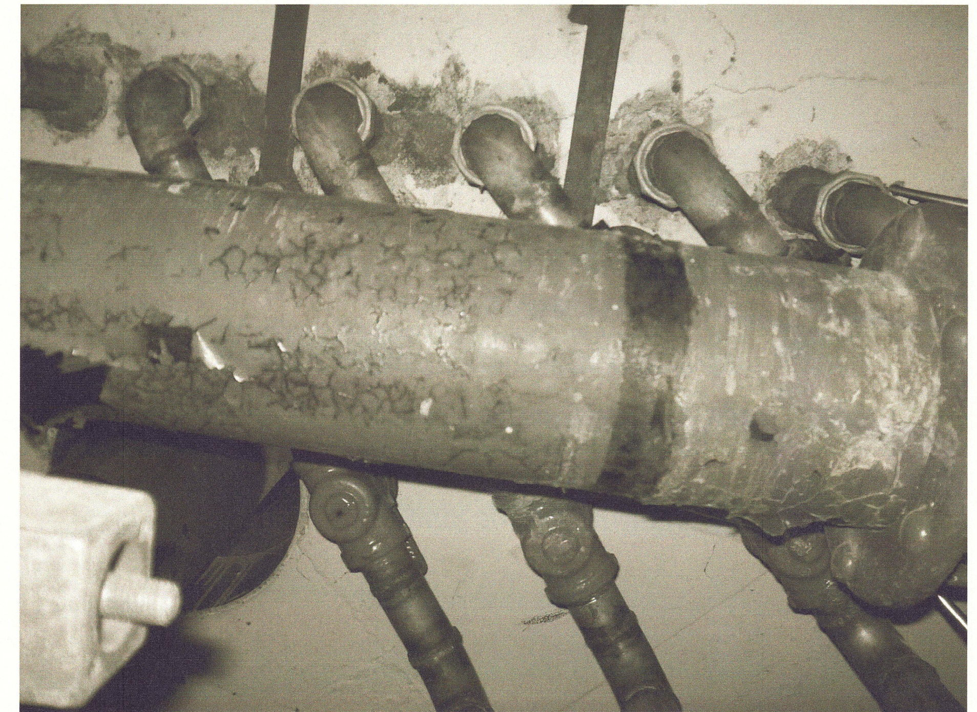
EXISTING LOWER LEVEL GAS FEED PIPING NTS
