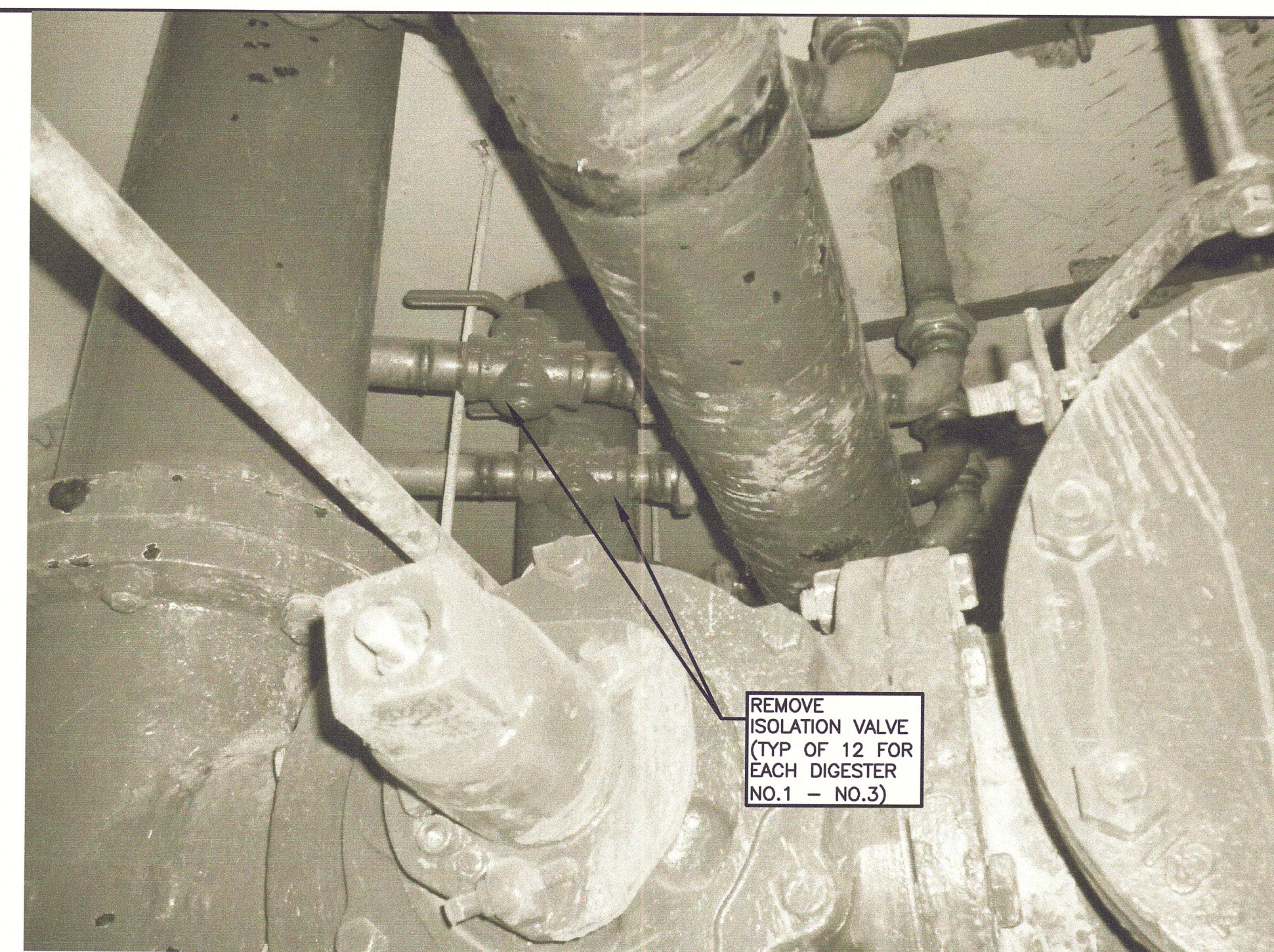
EXISTING GAS FEED PIPING NTS
