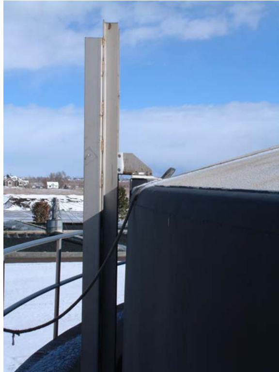
Figure 6. First generation slide guide assembly installed in digester cover.
