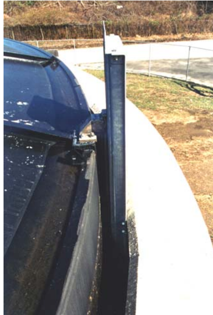
Figure 8. Full-length slide guide installed in digester cover.
