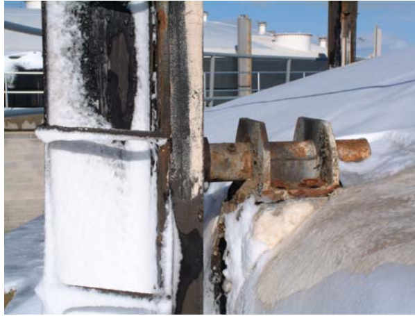
Figure 2. Roller guide installed on cover.
