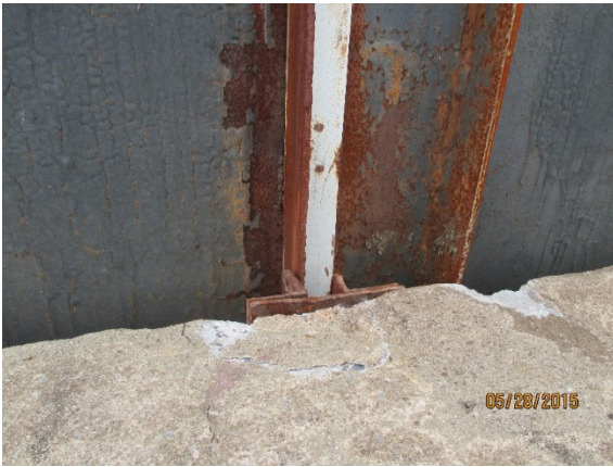
Guide C-D, Position 2 (Spalled Concrete)
