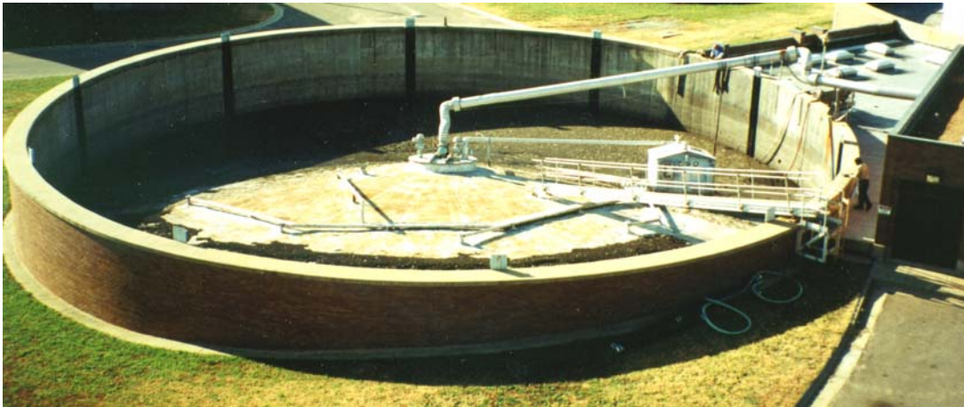
Figure 1. Tipped digester cover.
