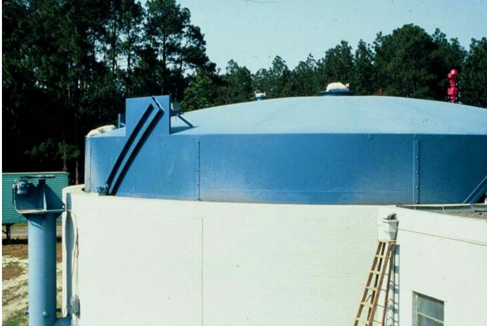
Figure 4. Spirally guided digester cover with rollers.
