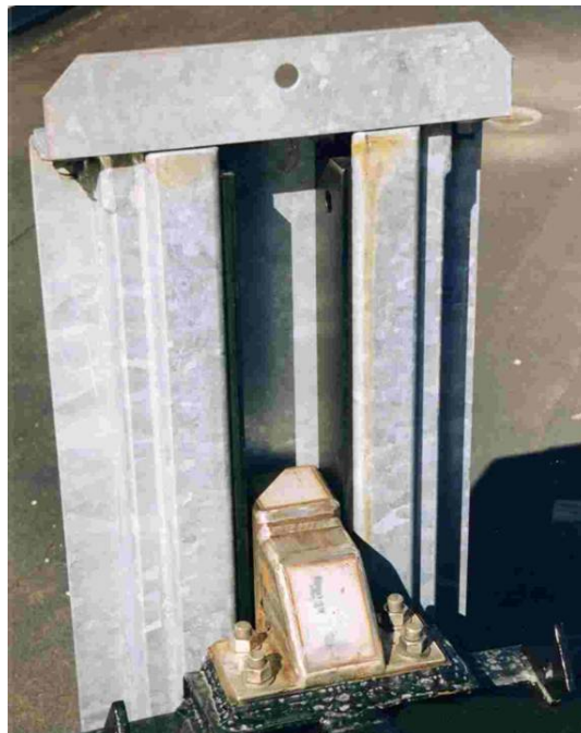
Figure 9. Full-length slide guide detail. Note hole at top of wear strip to aid removal.
