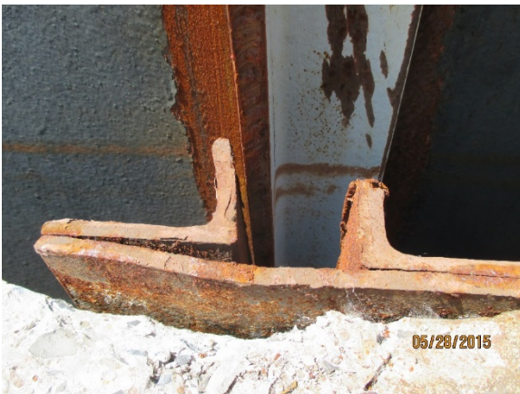
Guide C-D, Position 3 (Spalled Concrete & Bent Angles)
