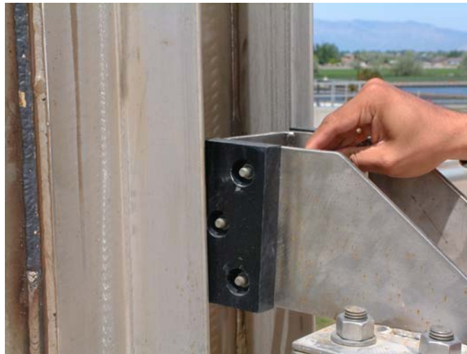
Figure 5. First generation slide guide assembly with UHMW wear blocks and stainless steel guides.
