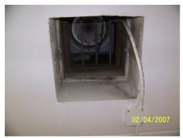
Vermiculite Mudded Thermal Insulation just below the Vent Fan Assembly
