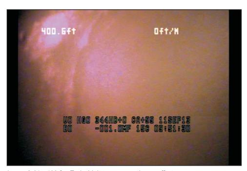
Image 3-06: 400 ft - Typical joint; no separation or offset
