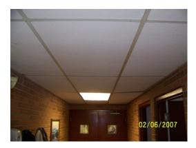
2-ft by 4-ft White Acoustic Ceiling Tiles Located in the hallway of the Control Building originally viewed as PACM by the NET 1991 Brewerton WTP Asbestos Survey
