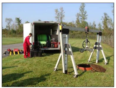
Figure 8: Manhole #12; Gantry with Metering Sheave
