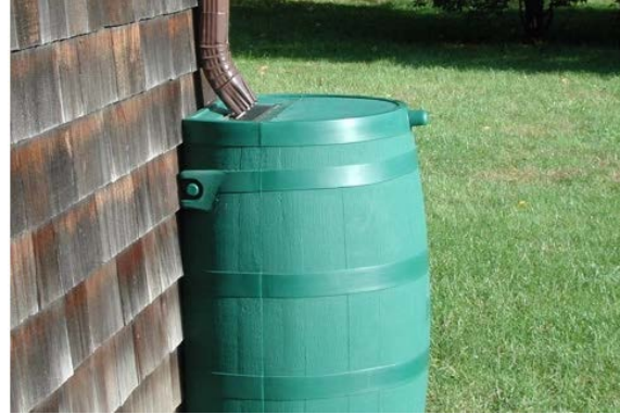
Rain Barrel Installation.
