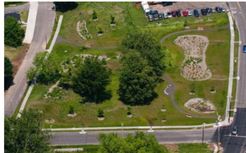
Green Infrastructure Facility Installed at the Intersection of Amy Street, Delaware Avenue and Grand Avenue.
