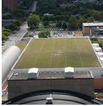
OnCenter Green Roof
