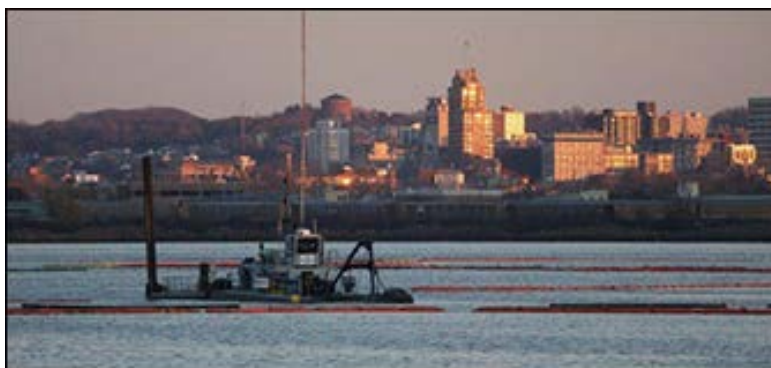
Dredging Operations in Onondaga Lake
