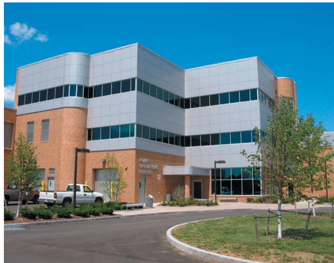
High Rate Flocculation and Settling (HRFS) Building
